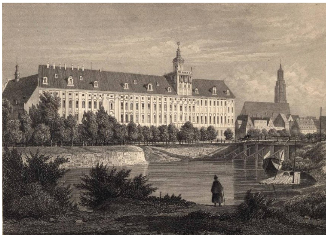
Figure 1. University of Breslau. Main building (19th century).
