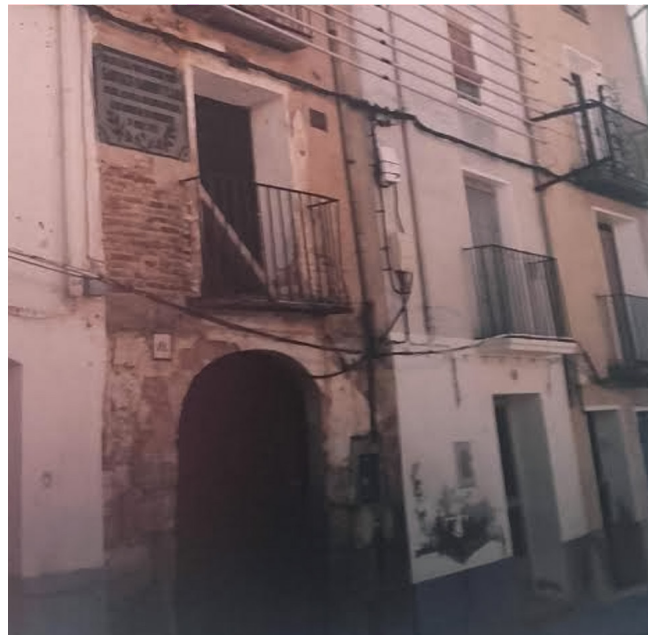
Figure 10. Above: Enriqueta Lewy posing in front of the Cajal family house in Ayerbe, where Santiago Ramón y Cajal spent his early years (1987; p. 164). Below: the dilapidated state of the building on 17 June 2018 (photograph by the author).
